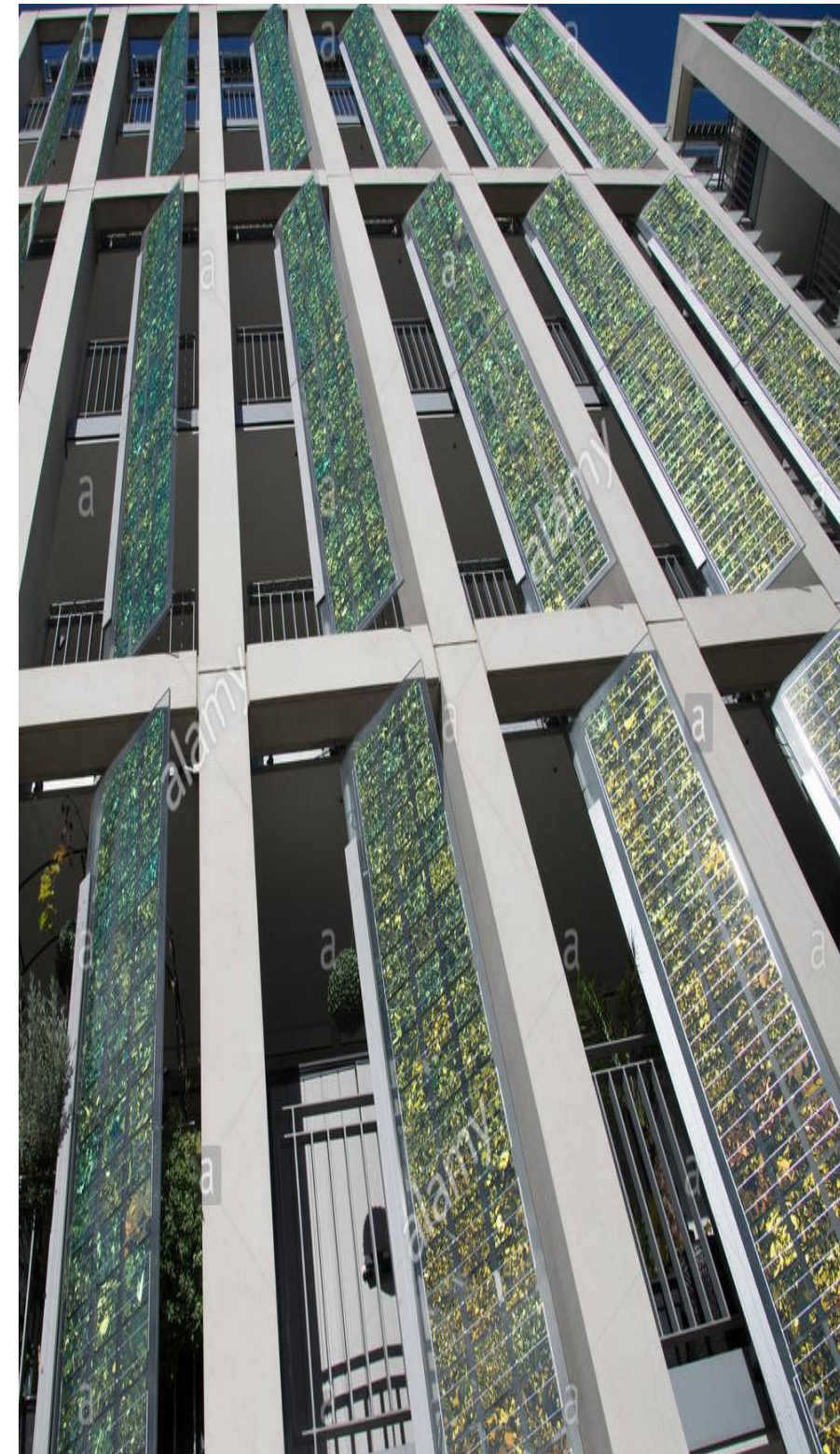
Solar shading device with horizontal overhang and vertical fins covered by non-reflective PV panel
