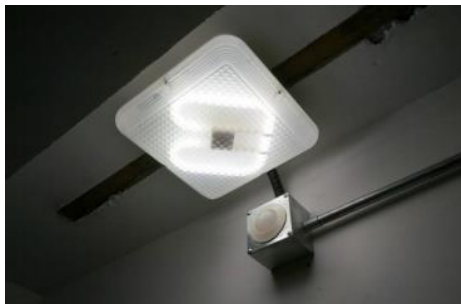
Motion sensor for lighting control (EMSD)
