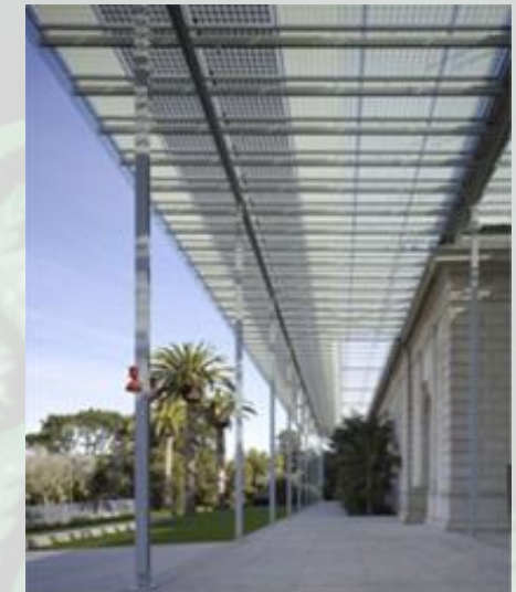
Reference example of integrated PV cells with the canopy in the California Academy of Sciences designed by Renzo Piano.
